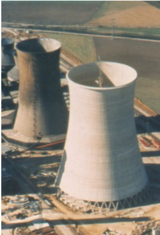
modern cooling tower R/t \gg 500
